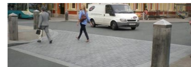
Figure 17. An example of how a courtesy crossing could be implemented at Moor Oaks Road, a busy side street along the travel corridor (Allianz, 2011)
